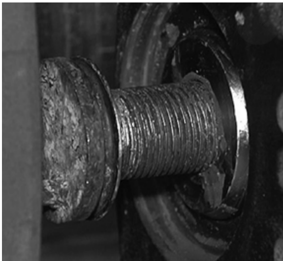
Figure 74: Corroded adjuster piston
