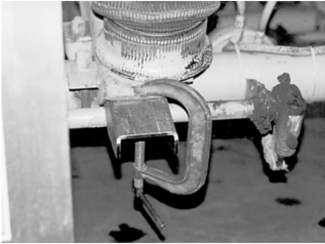
Figure 71: Temporarily holding beam extensions in place
