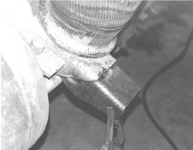
Figure 72: Tack weld rear beam extensions in place
