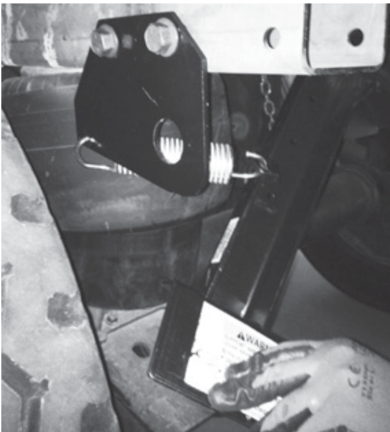
Figure 35: Arm raised above rail for spring installation
