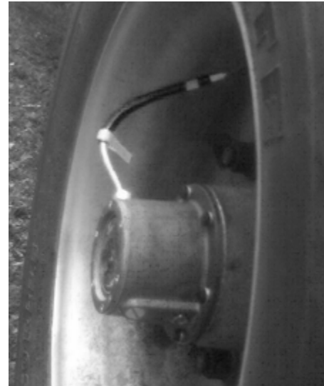
Figure 24: Sample tyre hose improper installation
